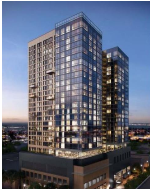
500 Main Street, New Rochelle, under construction as a residential building. Capital Prep proposes to house its charter school in this building
